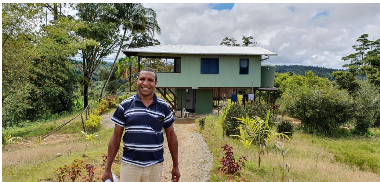
Head teacher of Kwiroknai Primary School Jonathan Kolda standing in front of the new staff house built by SDP funding received in 2018.
